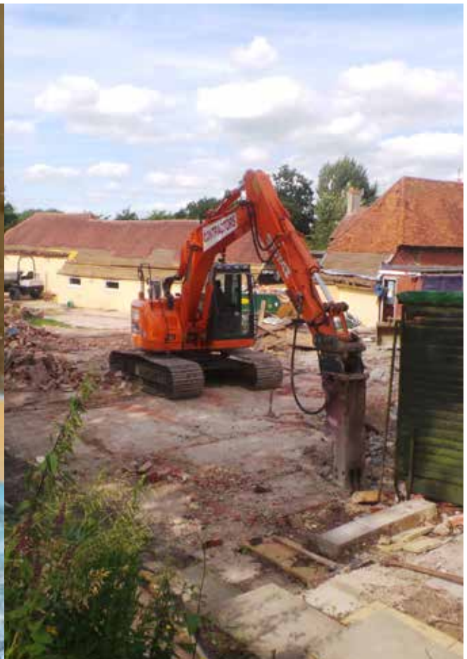
Our Newbury centre being rebuilt.
